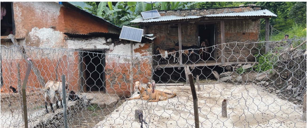
Improved Shed in Dullu Municipality
