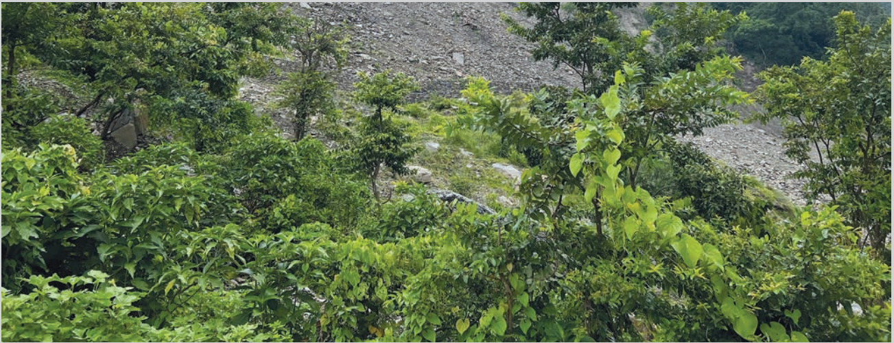
Slope Protection through Plantation
